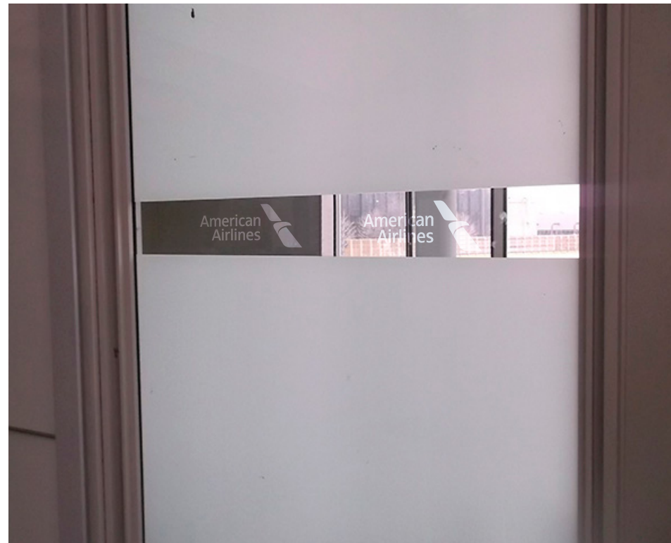
Admin Office over ATO, door glass, (After)
