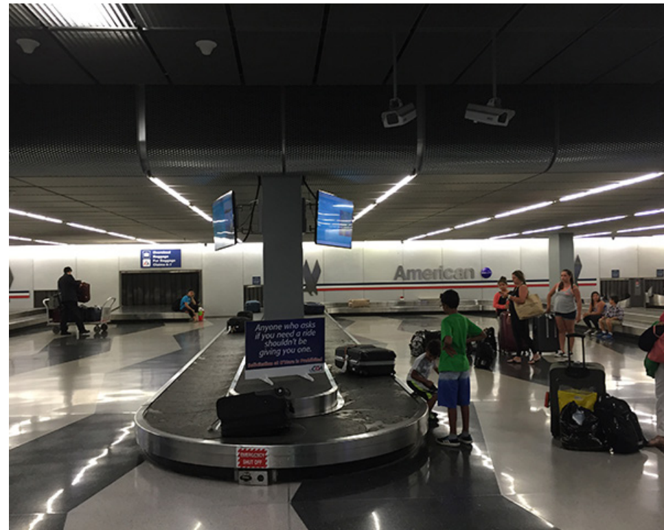
Baggage claim wall panel (LAA) behind conveyor 7 (Before)
